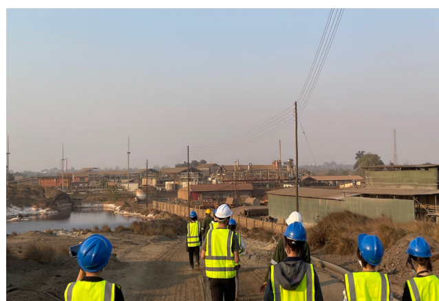
Fig.1 View of copper refinery at Kabwe
