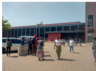
Kanyama General Hospital 外観
